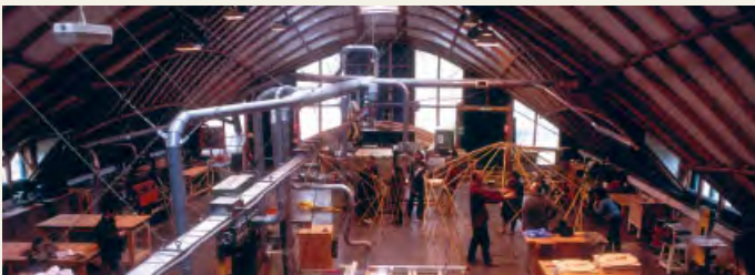
The interior of the workshop at Hooke Park, a structure based on a concept by Frei Otto and engineered by Buro Happold. The basket-like arches are composed of three sections of round wood, resin-spliced and bent into position whilst still 'green'. A concrete ring beam around the floor slab constrains the structure.
