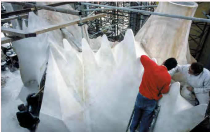
Full-scale mould-master for part of the central nave ceiling vaults (inverted for convenient fabrication at ground level). This plaster of Paris mould-master is for the production of fibreglass production moulds for building components.
