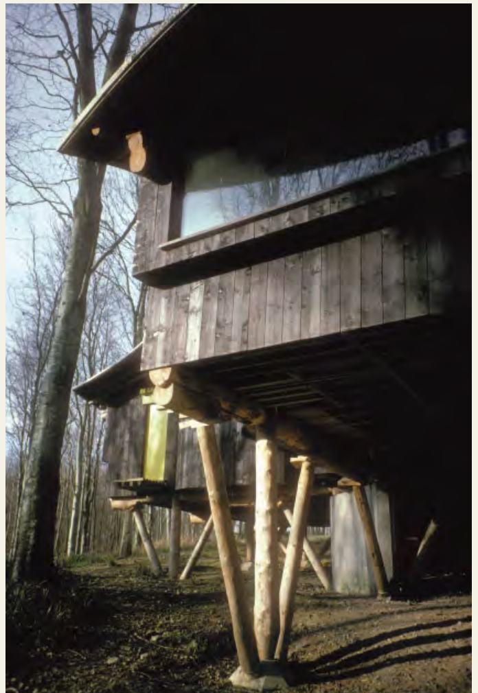
The Cullinan-designed accommodation block at Hooke Park. Adjacent are the footings for a fourth building that will be used to erect the first of the AA-commissioned structures.
