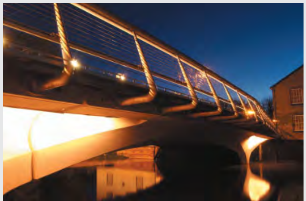
Ballingdon Bridge showing the illuminated scoops at twilight.
