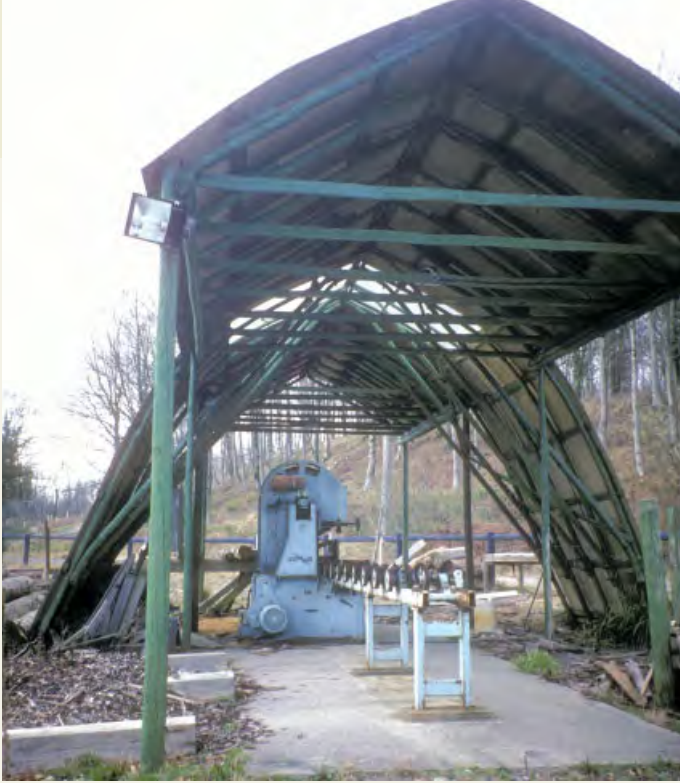
The simple structure shielding the circular saw at Hooke Park. Designed by students from the furniture school, it uses the material agenda of green round wood with intelligent simple joints to make a small, exemplary, useful building.
