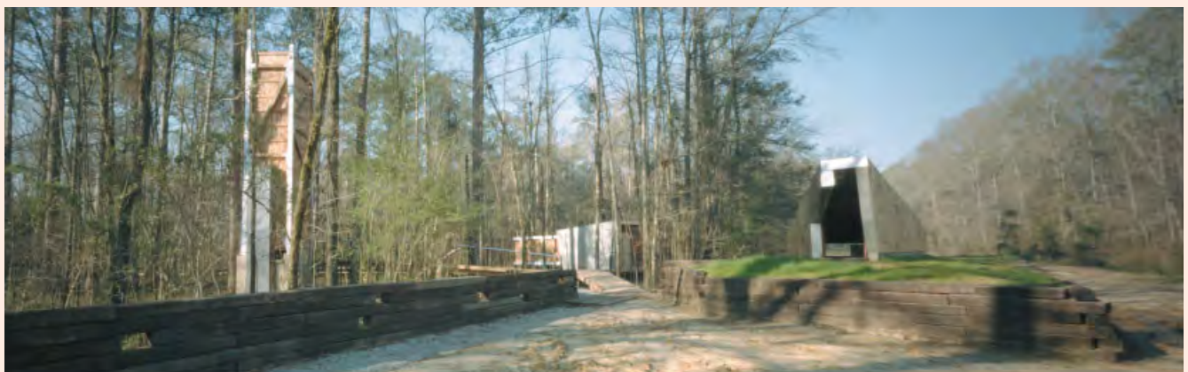
Perry Lake Park facilities, Perry County, Alabama, 2003 The park facilities were designed and built by Auburn University undergraduate architecture students Sarah Dunn, Matthew Foley, Brannen Park and Melissa Sullivan. Instructor: Andrew Freear.
