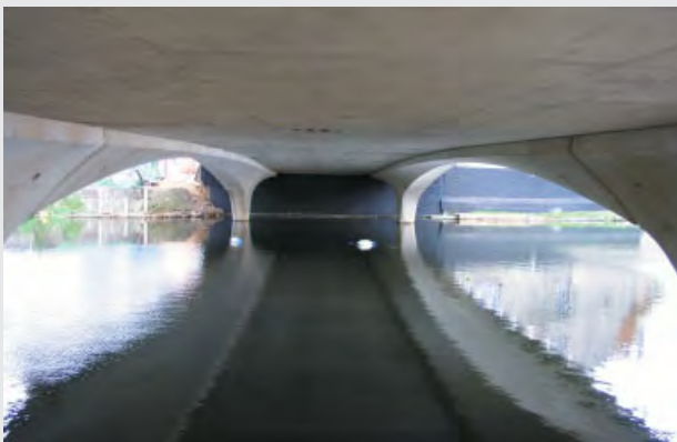
The in-situ reinforced concrete soffit of Ballingdon Bridge, including bat boxes. The in-situ concrete ties the precast concrete unit together to form an integral structure.
