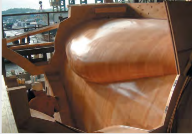
The Ballingdon Bridge pier mould showing the formwork of the scoops.
