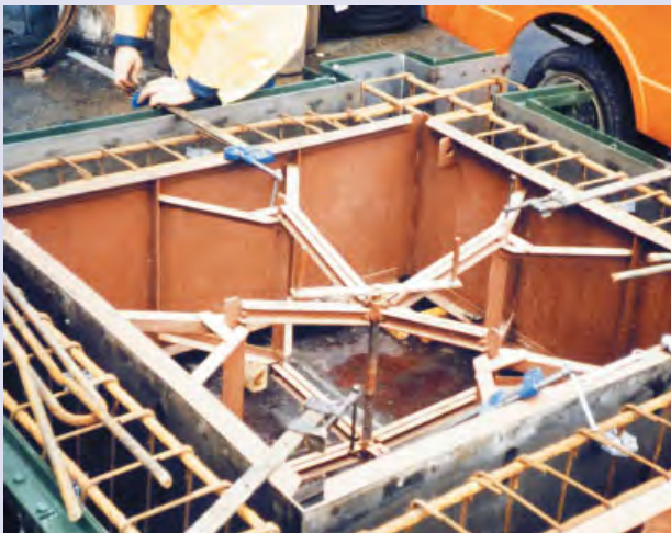
A prototype folding steel box form for the Lloyd's Building. Turning the screw in the centre of the box drew in the middle of the sides. This reduced the diagonal allowing the box to be withdrawn upwards.
