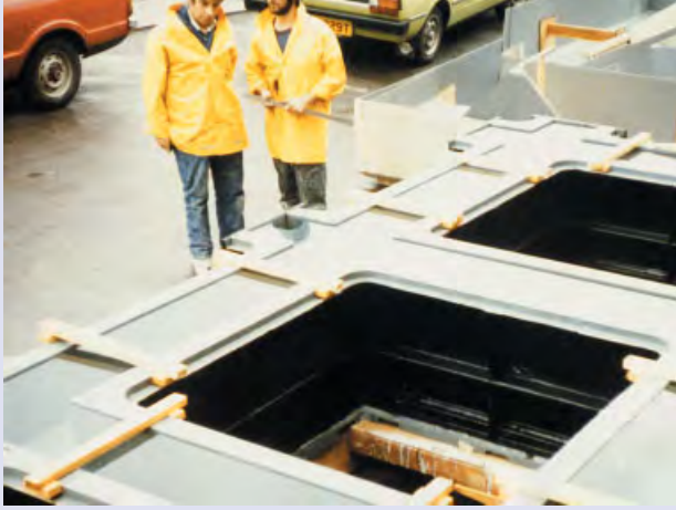
A prototype one-piece GFRP form for the beam grid of the Lloyd's Building. It was designed to be withdrawn upwards to avoid having the downward tapered beam profile of a conventional waffle floor.
