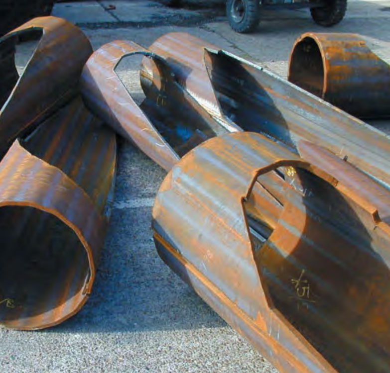
Figure 5: It fits where it touches. Prepared ends of the spikes prior to being interlocked and built as the core.
