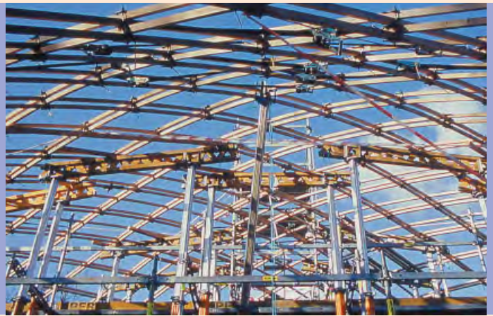
Support scaffolding and the gridmat midway through the forming process, showing the telescoping scaffold system in action.
