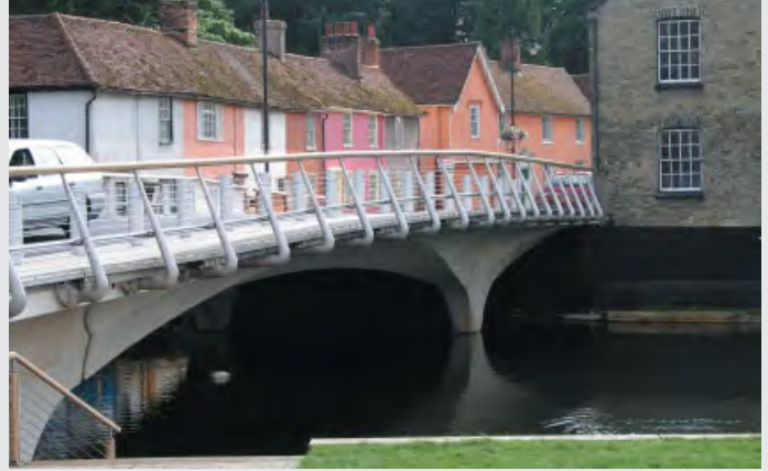
Ballingdon Bridge from the Sudbury bank.
