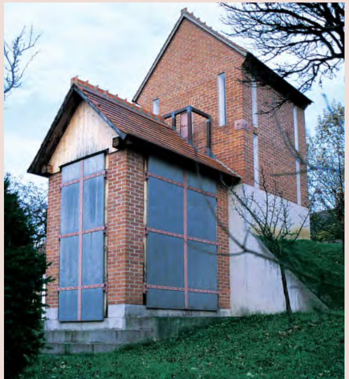
Small tower, Burgenland.
