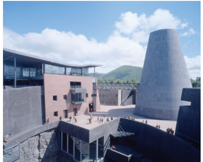
Hans Hollein, Museum of Vulcanology, Clermont-Ferrand, France, 2005 Architecture of the underground, looking down into the museum from ground level.
