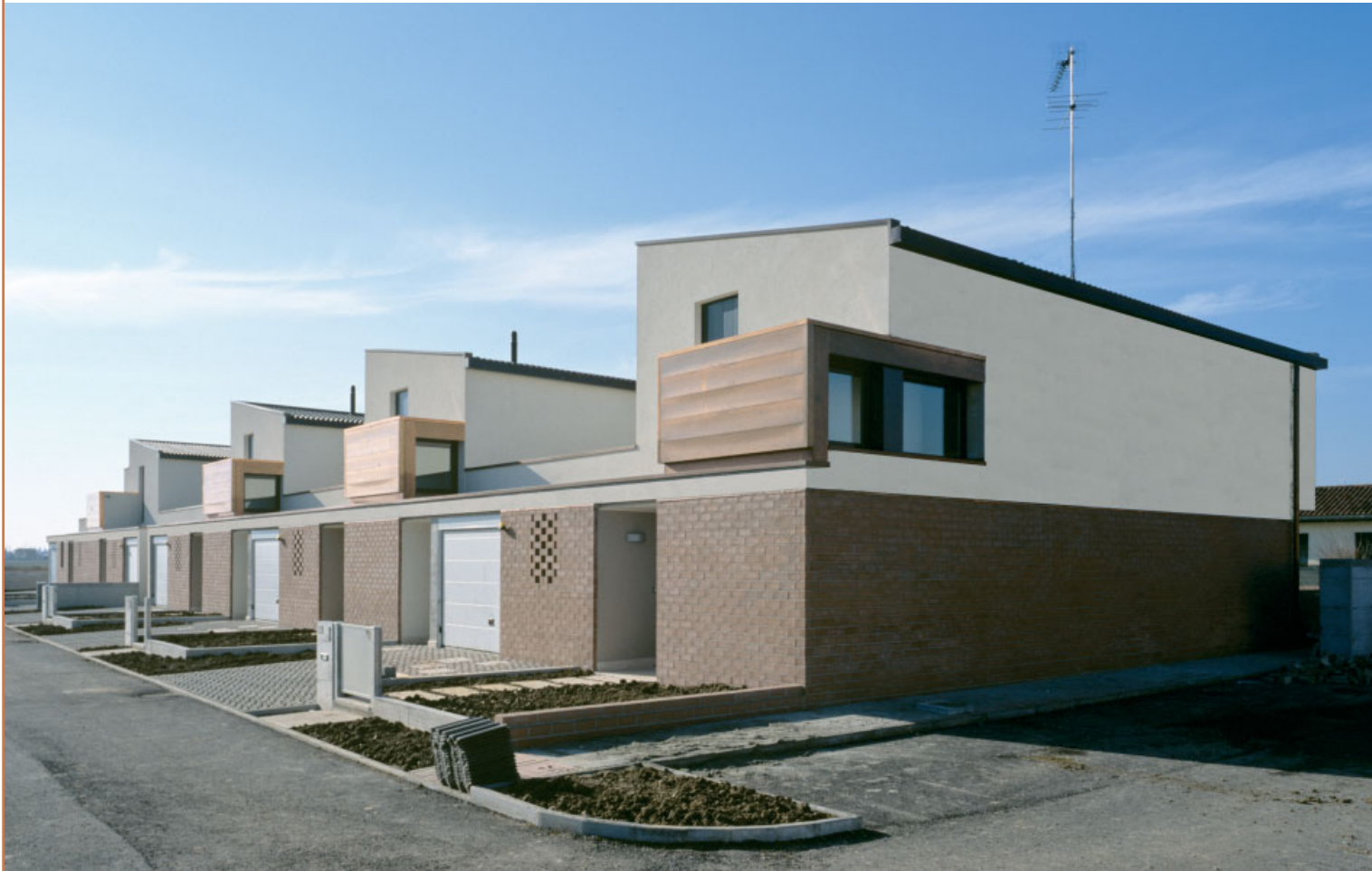
The two units of five houses that form the complex next to the countryside are unified by a continuous exposed-brick base, within which are set the garages and the entrances to the houses. A projecting structure, clad in copper, houses the stairs to the first floor.
