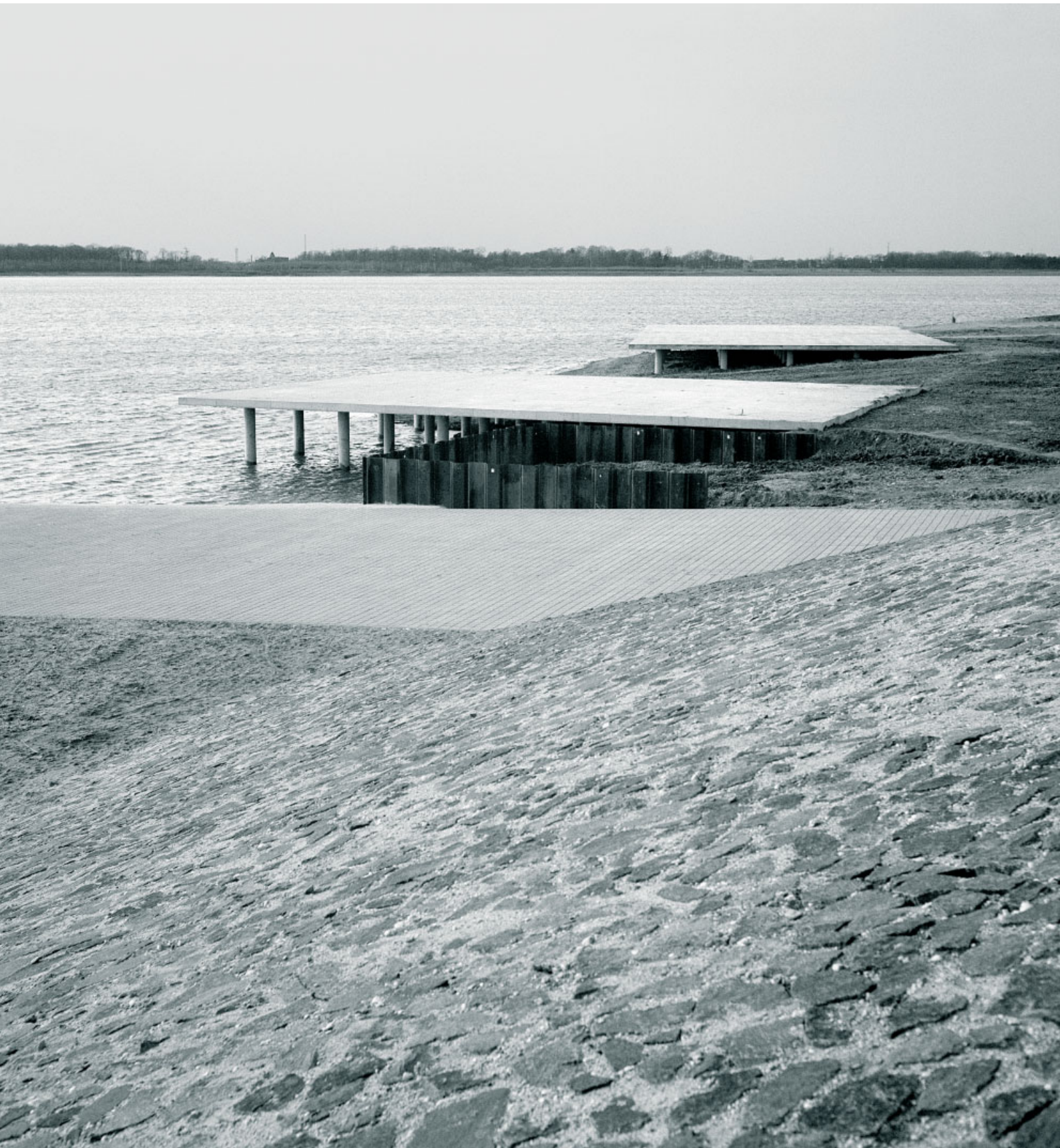
Structures on the new harbour ramp. The platforms emphasise the horizontality of the new landscape of lake and shore.
