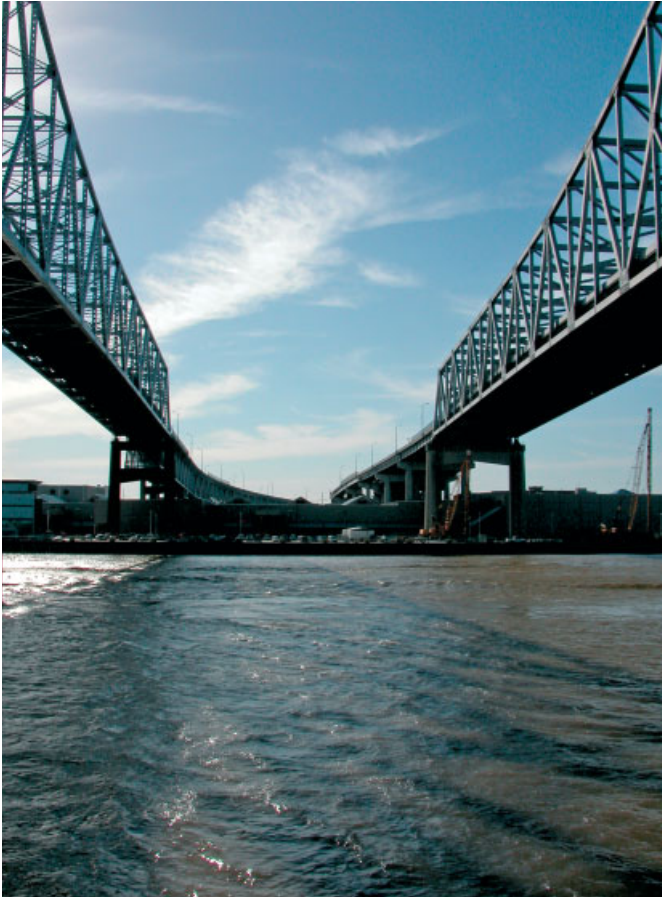
View of the freeway infrastructure from the river.
