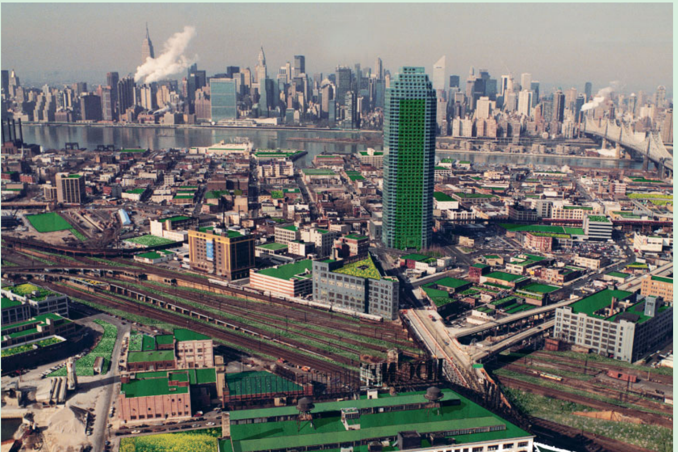
Balmori Associates, Green Roofs, Long Island City, Queens, New York, 2002–25
