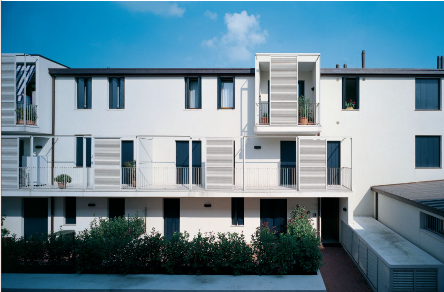
On the first floor of the subsidised housing complex, the facades are screened by continuous terraces and projecting balconies on the upper storey that are overlooked by the living spaces. Sunbreakers are used to create more privacy.
