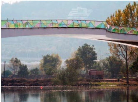
Figure 11. Arup AGU, Pedro and Inês Bridge, Coimbra, Portugal, 2007 View of the bridge from below, showing the 'cut-and-shift' forming the 'floating' square.
