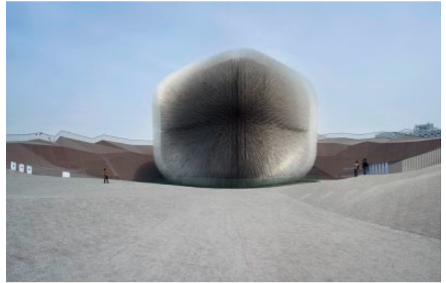
The pavilion is constructed from 60,000 7.5-metre (24.6-foot) long acrylic rods suspended in a timber frame structure.
