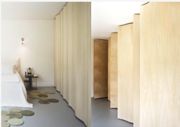
Figure 3. EZCT Architecture & Design Research, Seroussi Cupboard, 2005–8 The fully scripted panel system leads to an entirely automated fabrication process. The double-curvature surfaces of the panels are glued on to a light structure. Everything is built from standard and cheap wood with vertical T-shape steel reinforcements. The algorithms calculate the admissible deformation of the veneer wood (which is supposed to be close to zero) and propose different solutions. Due to very strict constraints, all stainless-steel hinges were conceived by EZCT.
