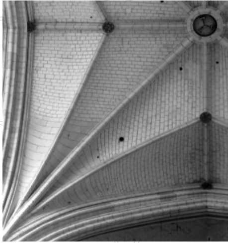
Figure 5. Amiens Cathedral, Amiens, France, 13th century left and opposite top: As systems of one logic are sequentially propagated along surfaces of a divergent logic, ruptures inevitably occur. Such ruptures are common in Gothic design, for example here in the vaults of Amiens Cathedral.
