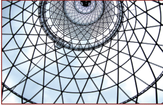
Figure 12. Vladimir Shukhov, Shabolovka (Shukhov) Tower, Moscow, 1922 Interior view showing a series of hyperboloids of revolution stacked on top of each other.
