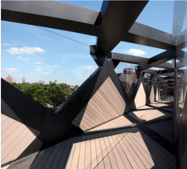
Figure 2. Arup AGU, Weave Bridge, University of Philadelphia, Pennsylvania, 2009 Interior view of the Weave Bridge with its interlacing steel structure and timber and glazed infill panels.
